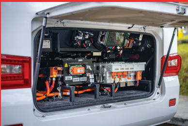
HIGH CAPACITY BATTERY 175 KWH
